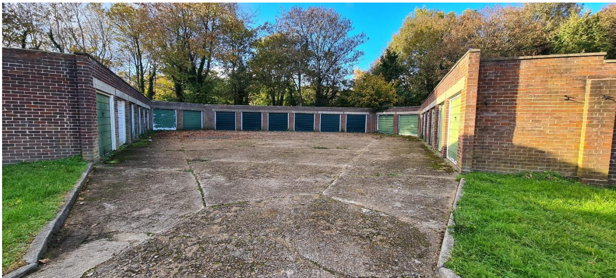
View of the existing garage blocks.
