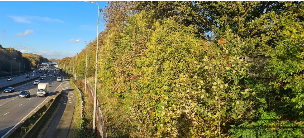
View of M25 showing it set at a lower level to the land on the right (beyond which sits the application site)
